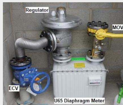
Figure 3. Diaphragm gas meter and fittings
