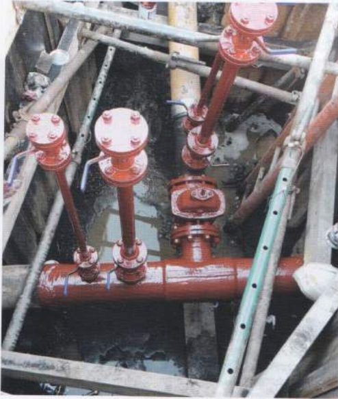
Gas pipeline connection work for Selby Power Plant
